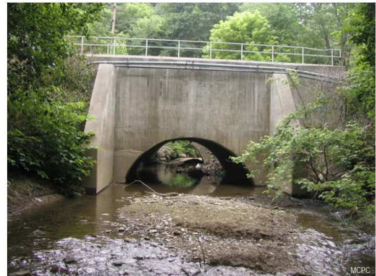
Railroad bridge over Gulph Creek in West Conshohocken
