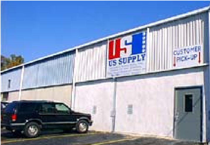
U.S. Supply on Portland Road is housed in an existing light industrial area.
