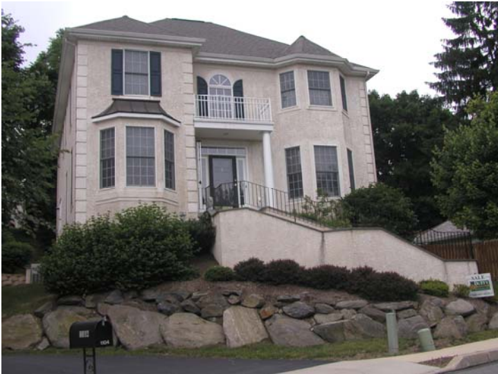
A modern house built in the Merion Hills neighborhood of West Conshohocken
